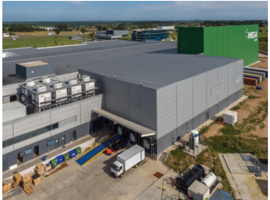
The loading and unloading docks are set off on their own to avoid interference between the two operations
