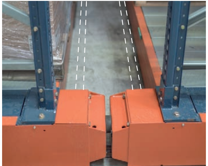
Interior safety barrier
