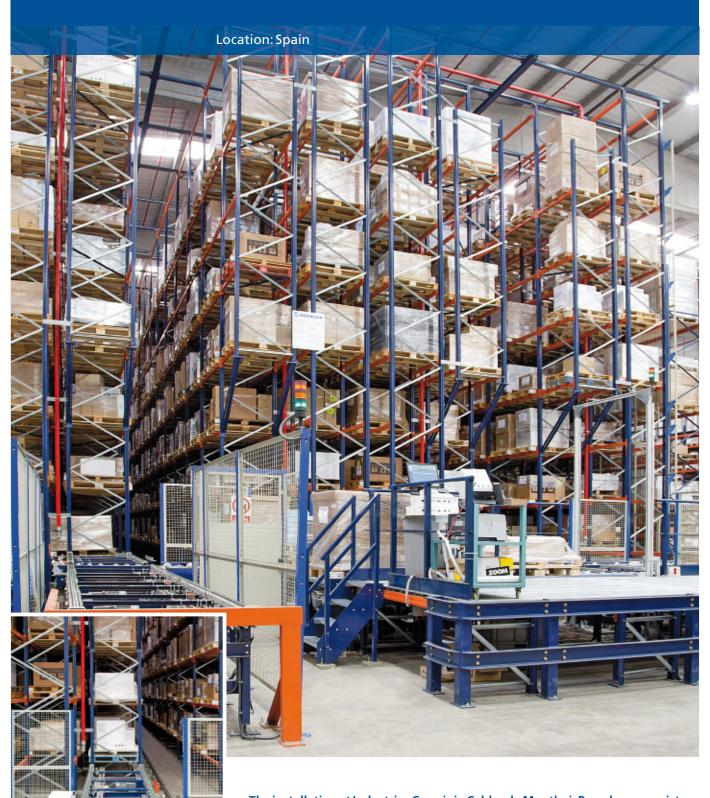
The installation at Industrias Cosmic in Caldes de Montbui, Barcelona, consists of an automated warehouse with live channels and a picking station at the front, plus a warehouse with adjustable pallet racking for bulkier products. The project included the Mecalux Easy WMS warehouse management system, responsible for managing all the activities carried out at the site.
