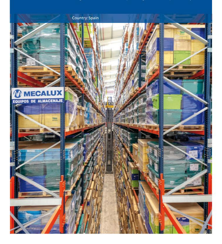
Francisco Martínez Piedras has centralised its logistics operations in two warehouses located next to its plant in Martos (southern Spain). Both have been equipped with narrow-aisle racks measuring up to 19 m tall, thus optimising both the surface area and height of the installation. Every day, a total of 7,500 SKUs are managed, while 18,000 car parts are dispatched in 1,200 pallets, which are then distributed to the company's customers in Europe, China and the US.
